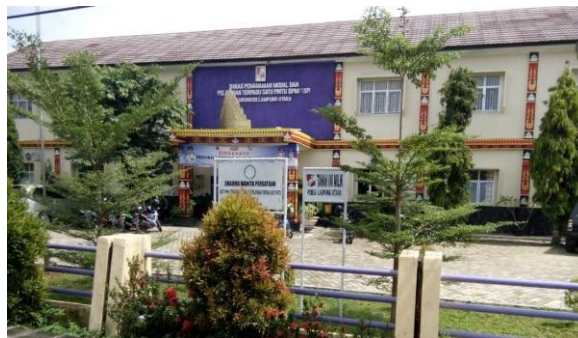
Figure 2. Office Building of the Department of Investment and One-Stop Integrated Services of North Lampung Regency placed here
